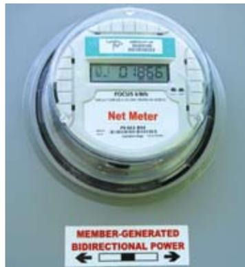
The net meter is designed to monitor the way electricity is flowing. When electricity is being generated by the PV system, the meter records the flow of it onto the co-op's system. At the end of a billing cycle, the meter is read to determine whether more electricity was generated than was used. Depending on the month, a bill will show an amount owed or credit earned.
