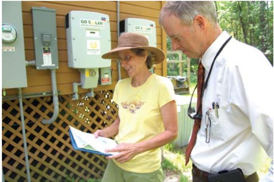
Co-op member Barbara Beck discusses her home's PV system with Sherman Phillips, Energy Services Manager for Clay Electric. Also shown are some of the components that make up the system. Shown, from left, are the net meter, the AC disconnect and the two inverters that allow the system to take the DC voltage from the panels and convert it to usable AC power.
