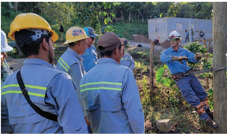
Lineworker Matt Hickey talks to the local municipal electric company workers about the project. At bottom, Hickey pulls line by hand.
